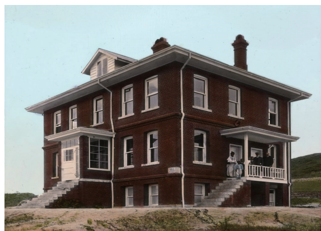
Fig. 2. Swedish Methodist Hospital (1913).
