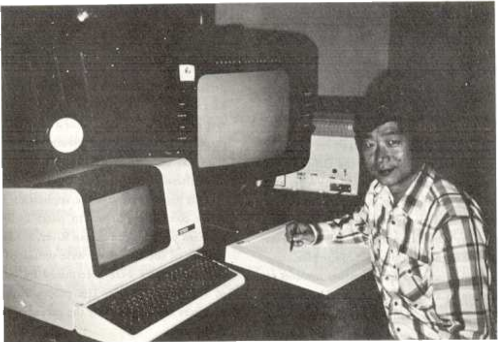
Fig. 1. Interactive Display Terminal, Digitizing Tablet and Pen (Cursor).
